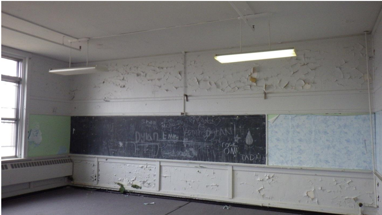
Typical Classroom Lighting
