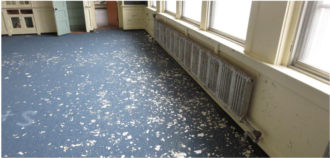
Typical Cast Iron Steam Radiator
