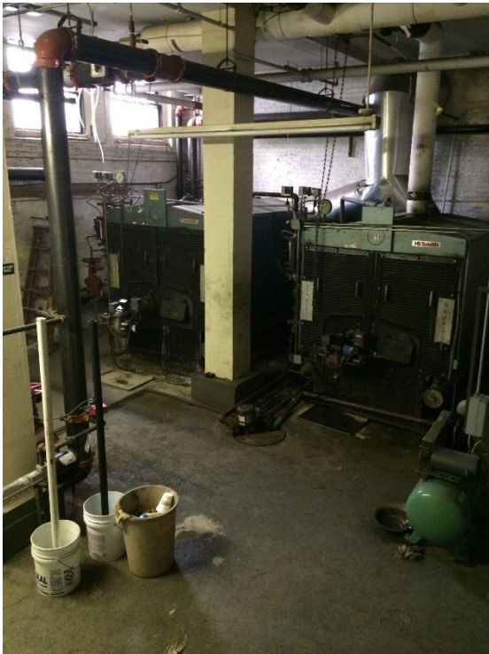
Cast Iron, Oil-fired, Steam Boilers
